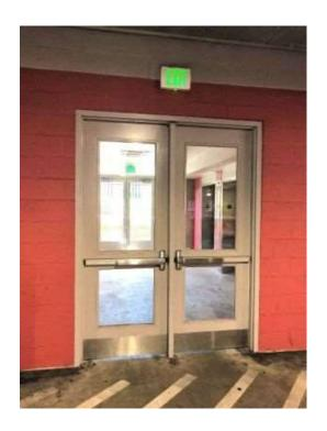
Swinging fire door assemblies protect openings in walls that are constructed to compartmentalize a building and resist the spread of fire. Without these fire doors as "opening protectives," fire-rated walls, partitions, and barriers with door openings would be unable to deter the spread of smoke, flames, and toxic gases during a fire.
