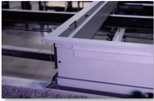
Bend tabs on jamb to lock to head
