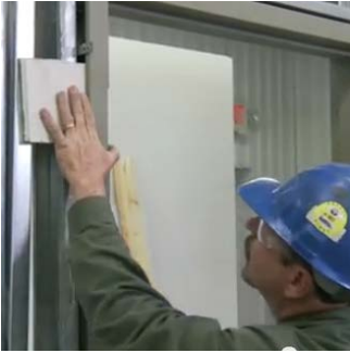
Attach to stud allowing for drywall thickness
