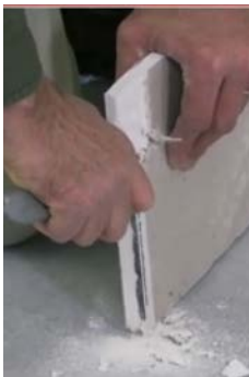
Chamfer back the edge of the drywall
