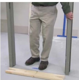
Stand the frame up in the wall line
