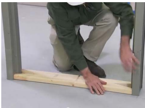
Place spreader between hinges and strike jambs
