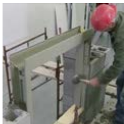
Tap the frames to settle the mortar
