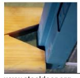
7. Insert a setting spreader at the floor of the opening. Make sure all four rabbets of the frame touch the spreader bar. This will prevent a twist in the frame.
