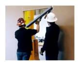
4. Slip the frame head over the rough opening header and center it in the opening.
