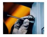
8. Snug the compression anchors evenly in each jamb. Use a level and a framing square to check for plumb, square, and twist.
